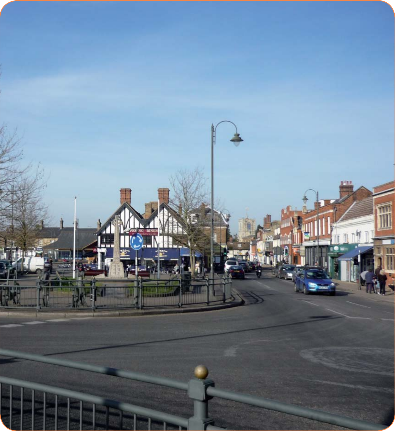
Figure 12/ Photograph showing how the junction between High Street and Station Road is dominated by vehicles with physical barriers preventing ease of movement for pedestrians
