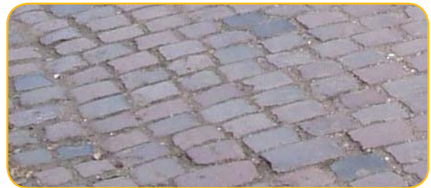
Granite Setts (eg Mill Lane)
